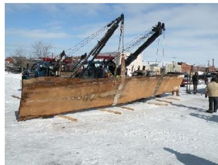
After arriving at Ancientwood's shop on a flatbed semi, the 40-foot board had to be lifted with cranes into an upright position. It was then lowered very carefully into a rolling-rack. Released from the crane straps, the board was ready to be wheeled into the warehouse. This beautiful solid slab is now on display in Ancientwood's warehouse until we find a buyer for it.
